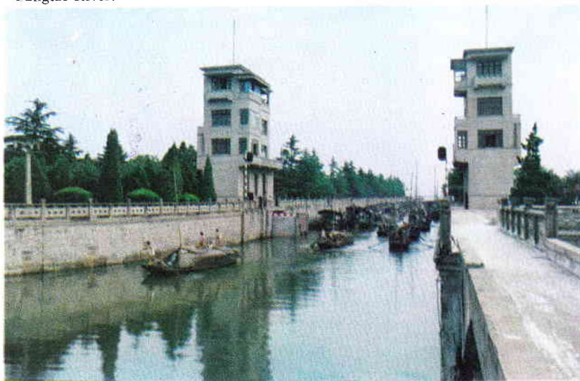
Lock at the exit to the canal enables ships to pass from its higher waters into the Yangtze River.
